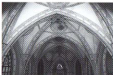
Fig. 3. The mural paintings and decorated plaster on the rib vaults in Clara church. Photo: A. Henningson
